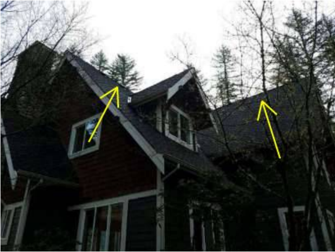
Photo 6-1 North side of home
