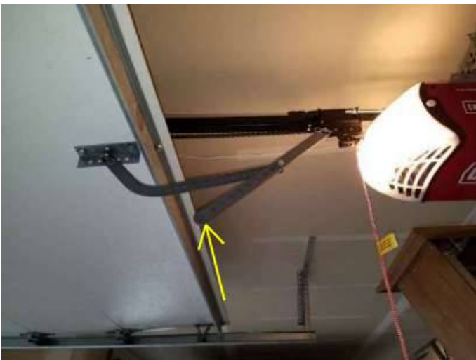
Photo 31-1 Missing bolt
