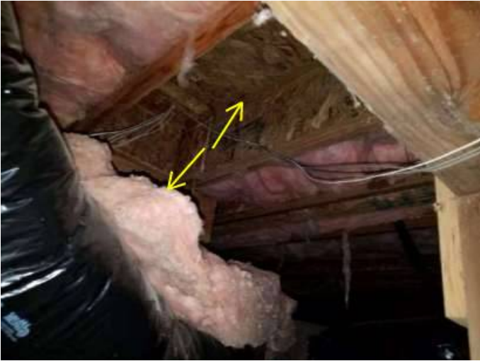
Photo 9-1 Living room area
