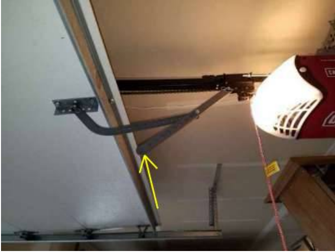
Photo 31-1 Missing bolt
